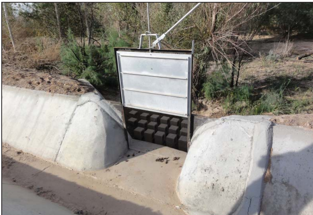
PHOTOGRAPH 4 Manually Operated Diversion Outlet
