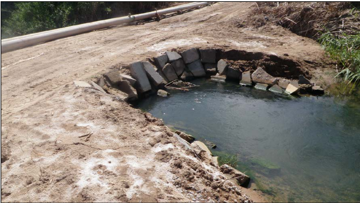
PHOTOGRAPH 9: Detail of a makeshift culvert crossing jurisdictional wetlands in central grubbed area.
